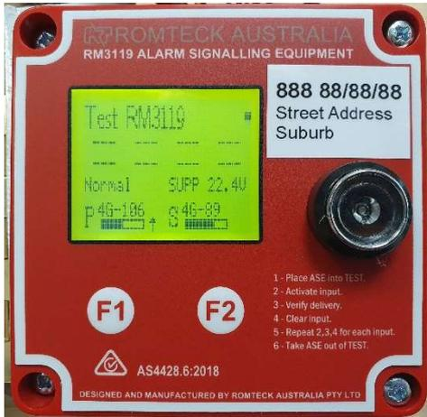
Image: An ASE RM3119 in Normal mode with no active alarms
