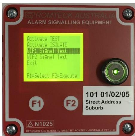
Image: Selecting WIP1 Signal Test
