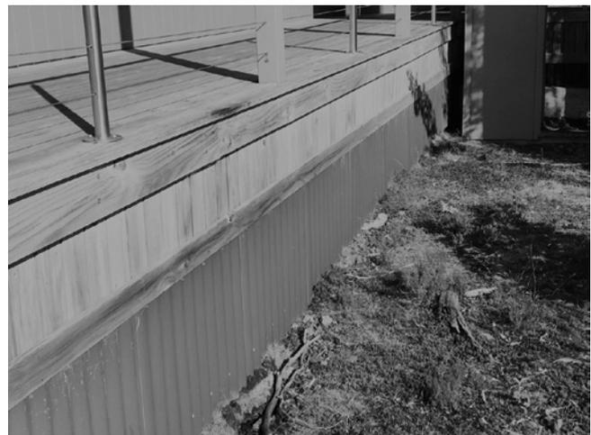
Examples of a simple building shape, simple roof design and an enclosed subfloor space on a deck
