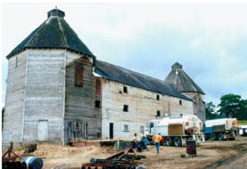
Remaining kiln adjacent to fire scene. Ignition point at 3 rd floor left window. Left vent also caught fire.
