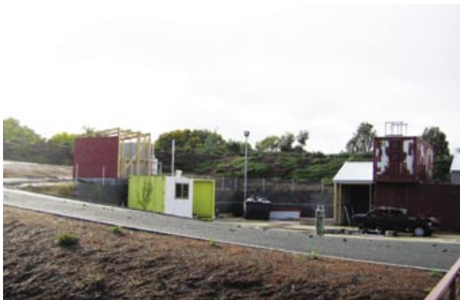
Changes to our gas prop facility and additions to the structural firefighting prop.
