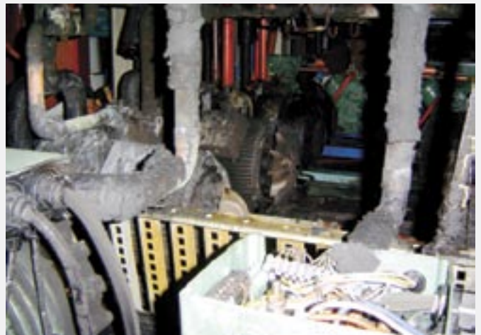
View of compressor bank - point of origin last unit on left hand side
