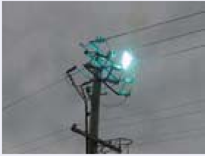
Power pole fire in Barton Street, Mowbray. Submitted by Firefighter Launceston Brigade, David Ransome
