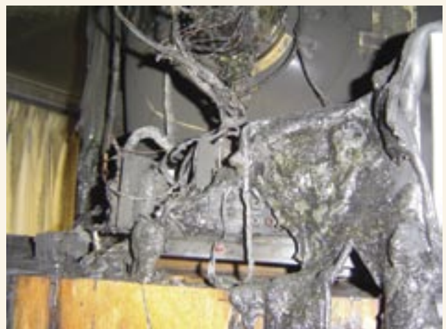
Rear view of TV from an unrelated incident. Cause - malfunction within TV set
