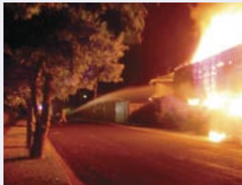
Ulverstone Grandstand fire on 12th January 2005 at 1.03 am. approximate damage $500,000.
